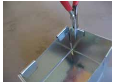
Set the braces into place and crimp with pliers.
